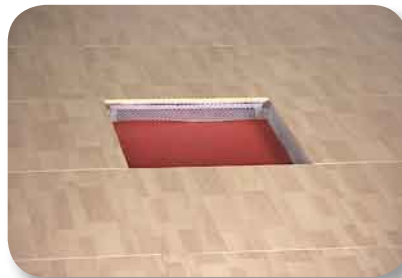
Space below the floor
